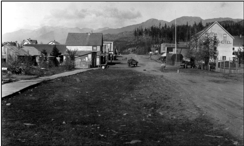
Figure 2. Terrace in 1920 on Kalum St, looking North.
