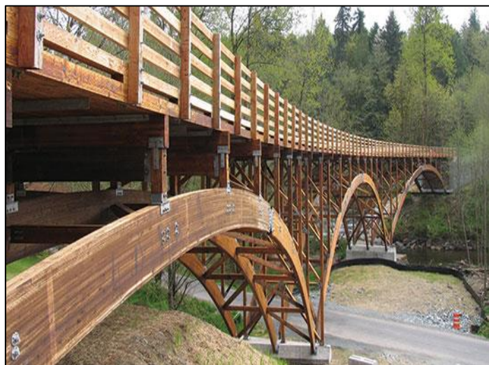
Figure 23. Bridge construction with glulam and other wood products.
